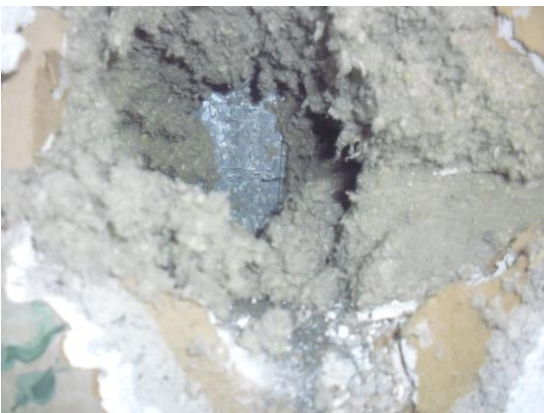
Floor 1 Room 3 Unwrapped Riser
