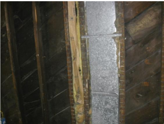
Floor 1 Room 1 unwrap riser
