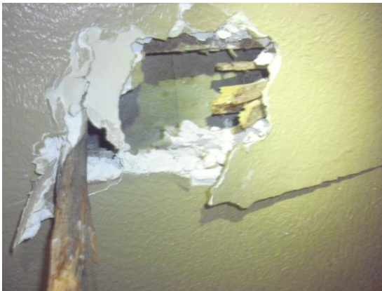
Floor 1 Room 3 Wrapped Riser
