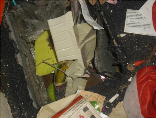
Floor 1 Room 3 Unwrapped Riser
