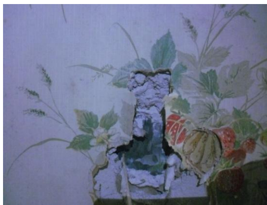
Floor 1 Room 2 Unwrapped Riser
