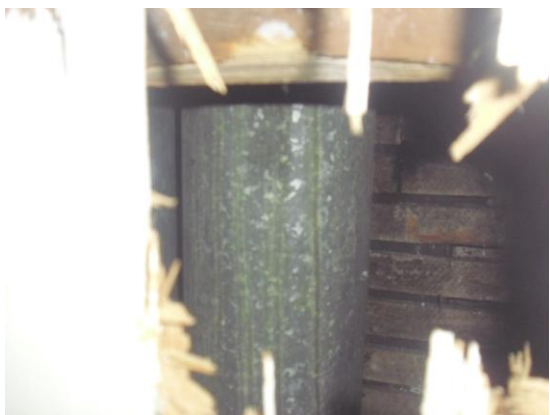
Floor 1 Room 2 Unwrapped Riser
