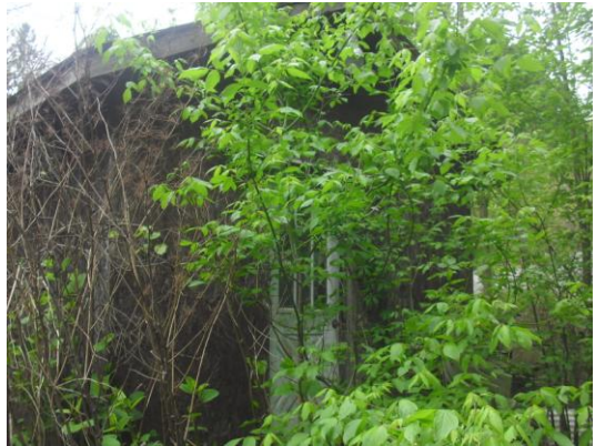
North Shed 2 Exterior
