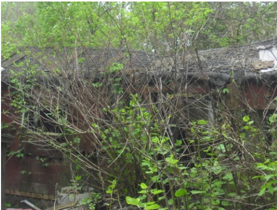
North Shed 1 Exterior
