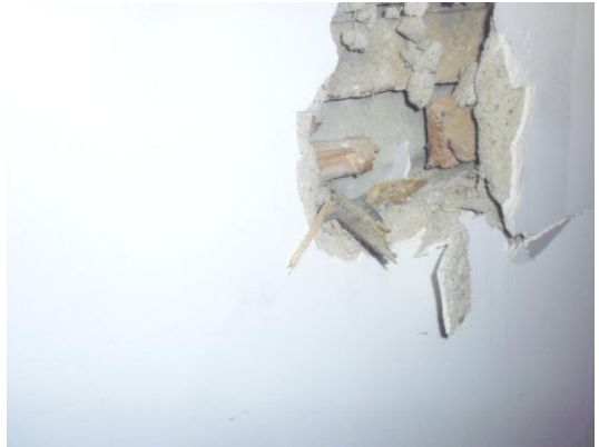
Floor 1 Room 2 Wrapped Riser
