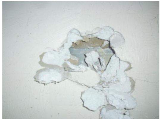
Floor 1 room 2 Unwrapped Riser
