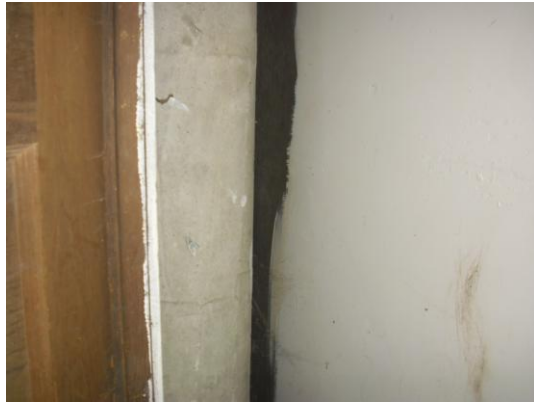
Floor 1 Room 3 wrapped riser
