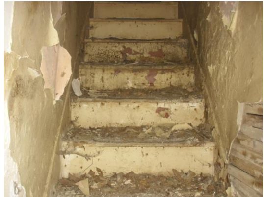
Stairs to Floor 2
