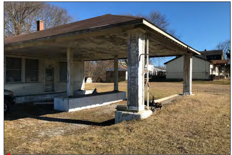
Photo 6: View of former dispenser island facing to the east.
