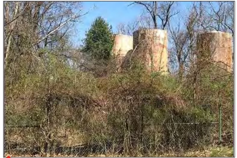
Photo 10: View of ASTs from south parcel looking north across Sulphur Run.
