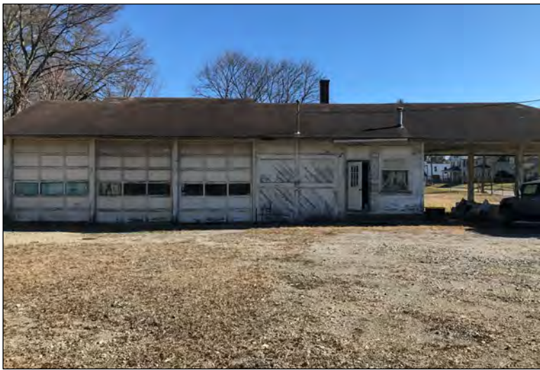
Photo 1: View of the garage facing east.
